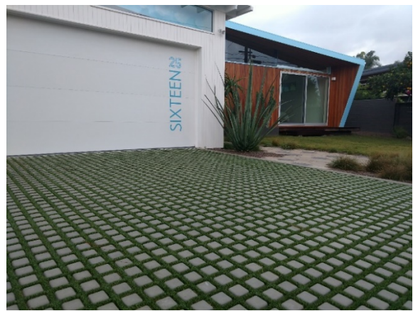
Photo 12: Finished Drivable Turf® installation
