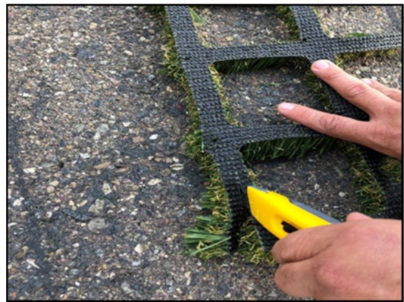
Photo 6: Backing cut for an edge termination
