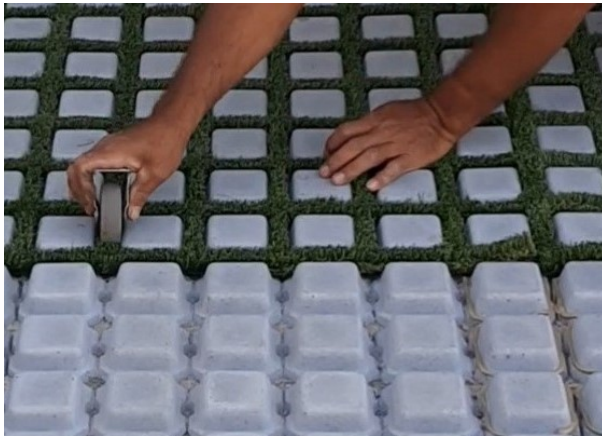
Photo 9: Wheel used to adhere turf
