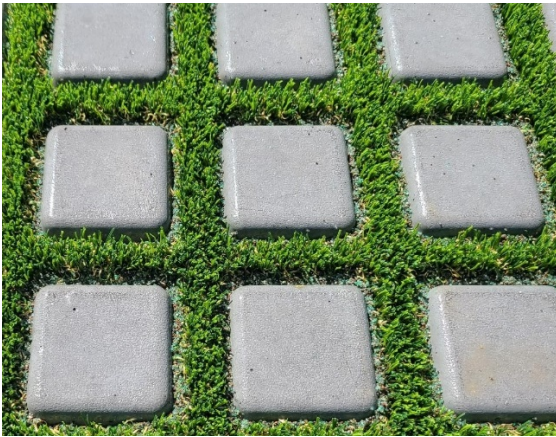
Photo 11: Finished installation using colored sand
