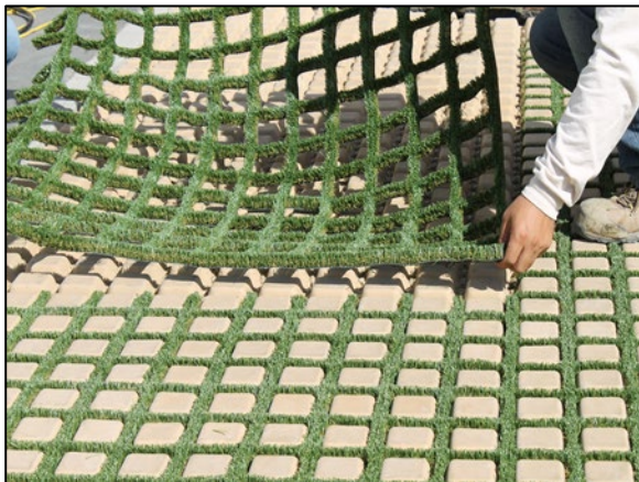
Photo 5: Pre-Fit Installation of Drivable Turf.
