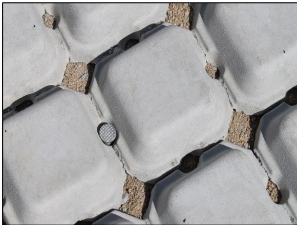
Photo 3: Spike driven into base of mat.
