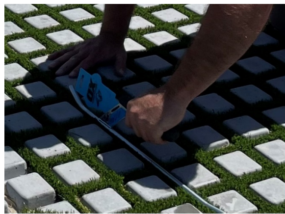
Photo 10: sled brick jointer used to adhere turf
