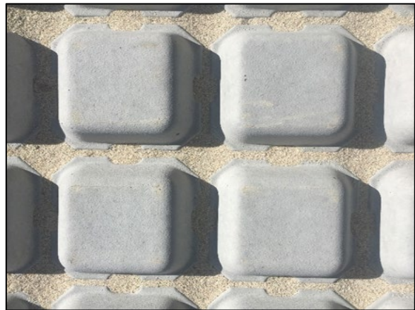
Photo 4: Sand filled to base of Drivable Grass mat
