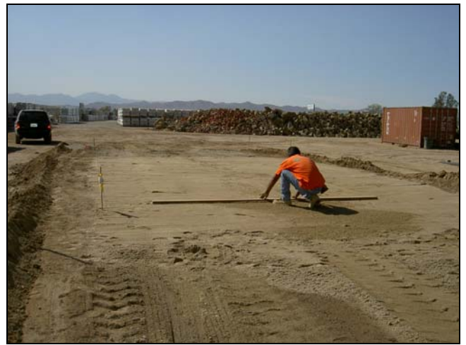
Photo 2 – Leveling Sand Bed Over Compacted Base
