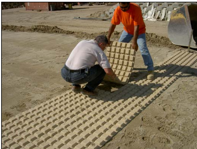
Photo 3 – Installation of Drivable Grass
