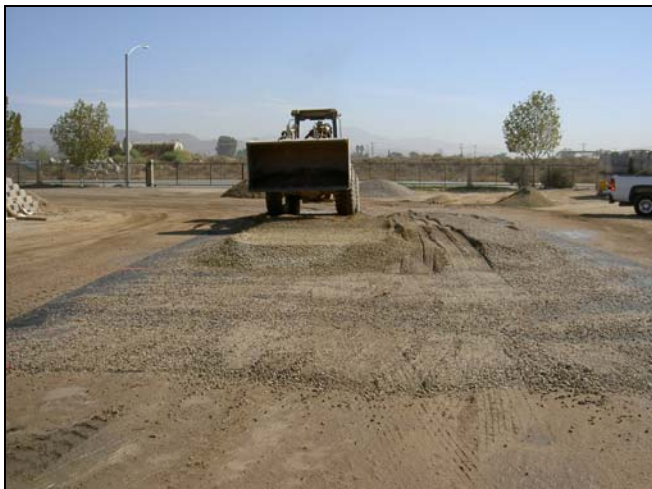
Photo 1 – Placing CMB Over Geotextile
