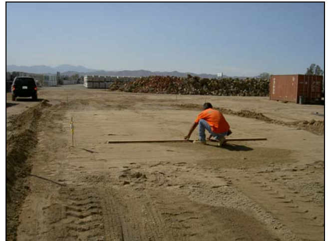
Photo 2 – Leveling of sand bed over compacted base
