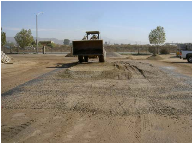
Photo 1 – Placing CMB over geotextile
