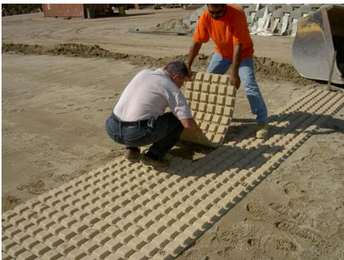
Photo 3 – Installation of Drivable Grass ®
