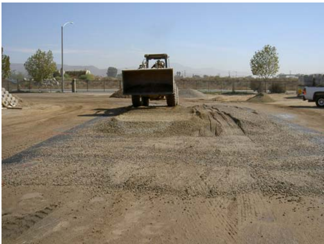
Photo 1 – Placing CMB over geotextile
