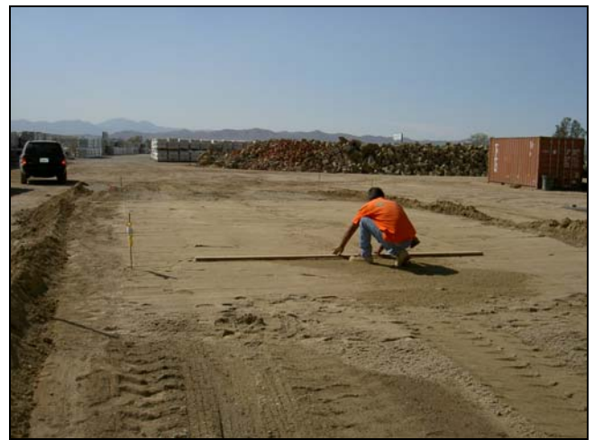
Photo 2 – Leveling of sand bed over compacted base
