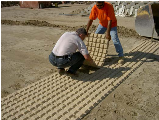
Photo 3 – Installation of Drivable Grass
